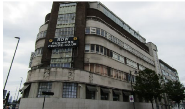
Fig. 15: Bow House Business Centre
